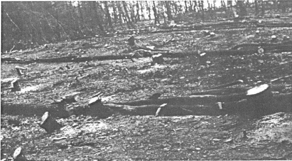
PHOTO 1. Construction of log-erosion barriers using felled burnt pine logs.
