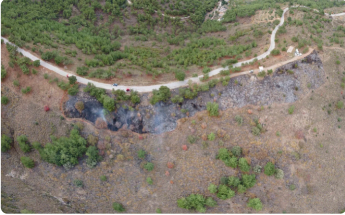
Treating and extending a shaded fuel break with prescribed burning. Author: Andrea Bonetti | © Educational use, non-commercial.
