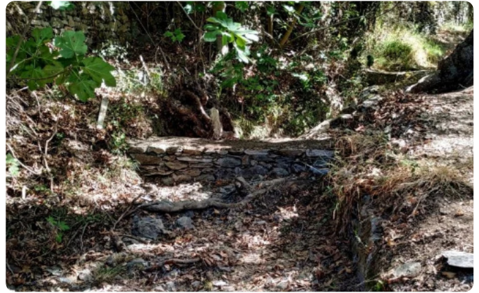
Completed micro-dams ready to receive water
