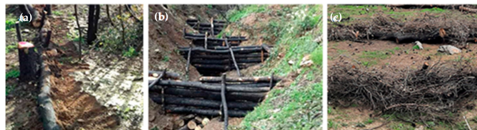
Figure 4. Different types of erosion control structures: (a) log barriers, (b) log dams, and (c) wattles.
