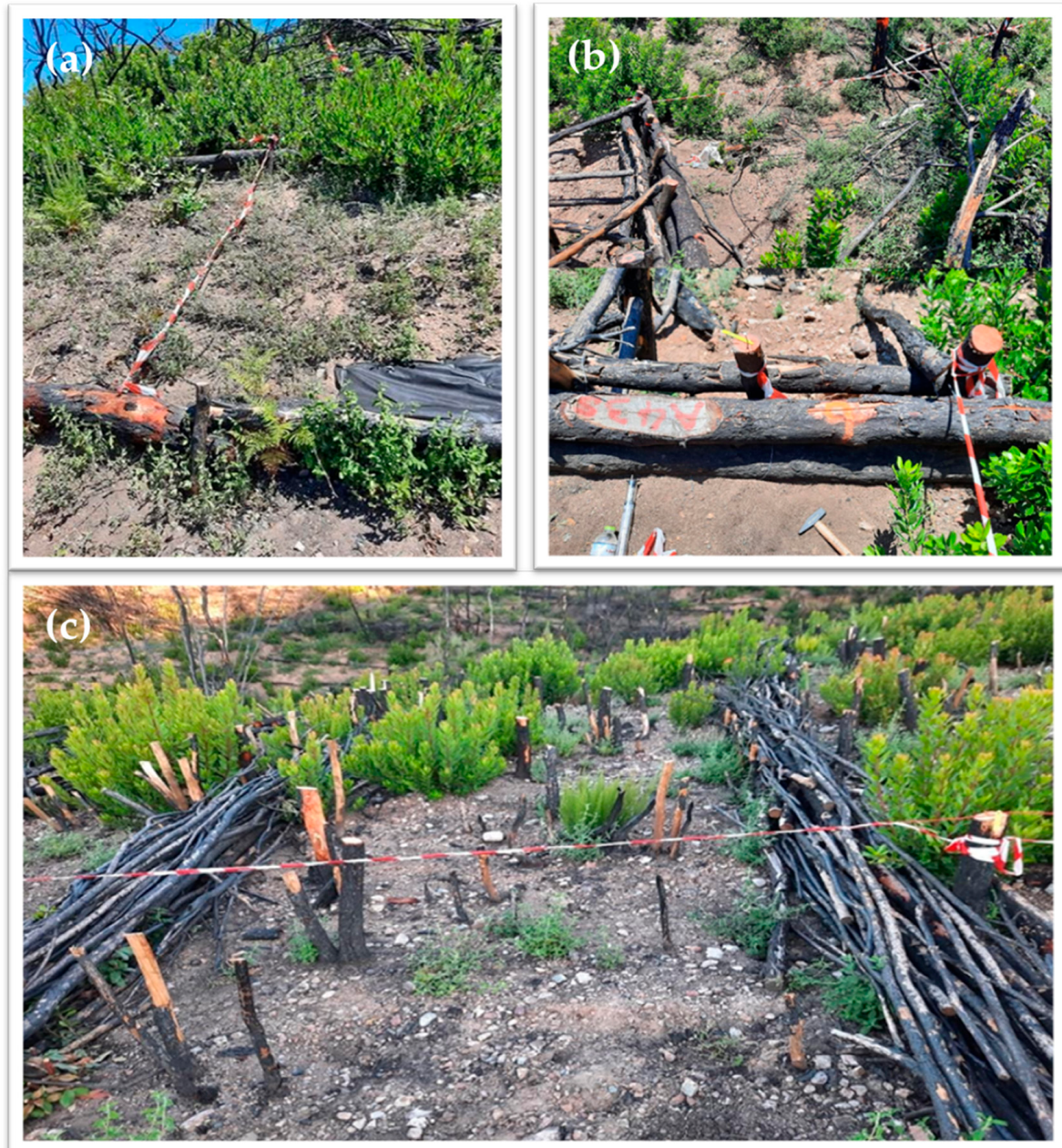
Figure 2. Different types of erosion-control structures: (a) log barriers, (b) log dams, and (c) wattles.
